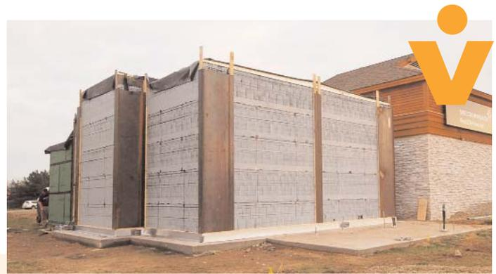
The use of individual VeriShield modules guarantee consistent density throughout the VPAC unit. It eliminates the potential for radiation hot spots caused by inconsistent concrete densities that may be found in modular concrete constructions.
