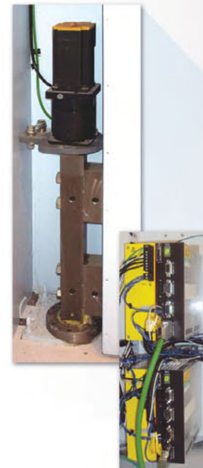
All motorized components and control box concealed behind panel on side of door—no loss of headroom.
